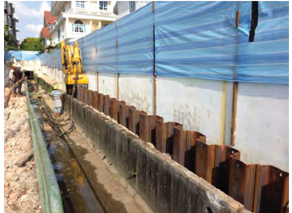
Press-in Method by Silent Piler
