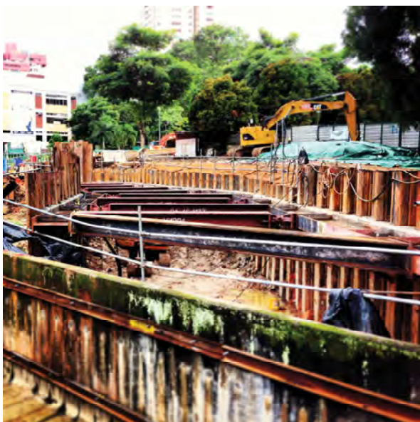
Temporary wall for Civil Excavation
