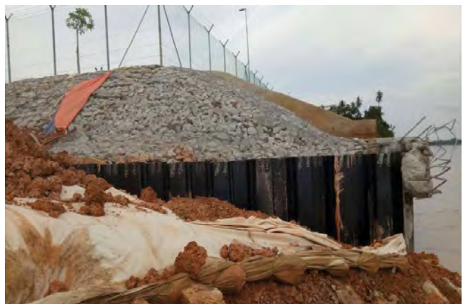
Permanent wall for Water Treatment Plant
