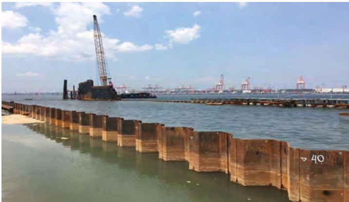
Quay Wall of Port Facilities
