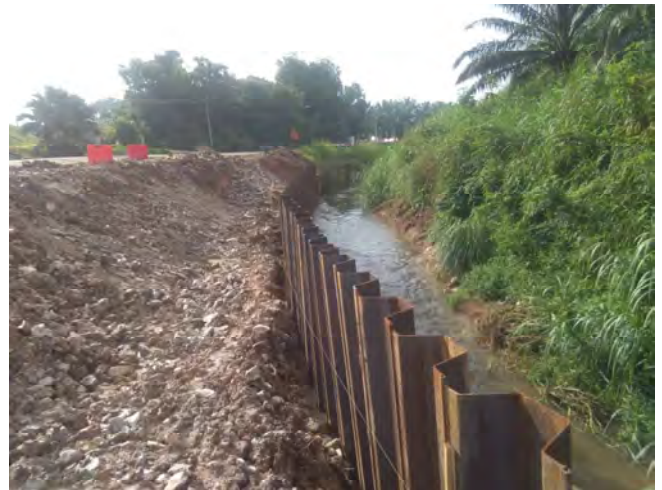
Flood Mitigation Project by JPS
